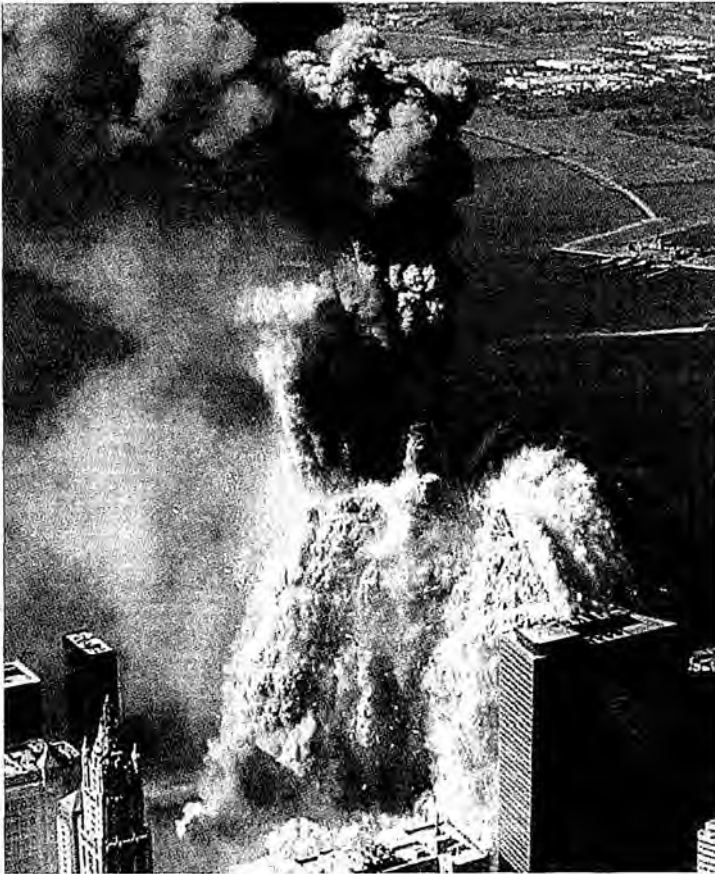
Figure 157. Does this look like a collapse?
