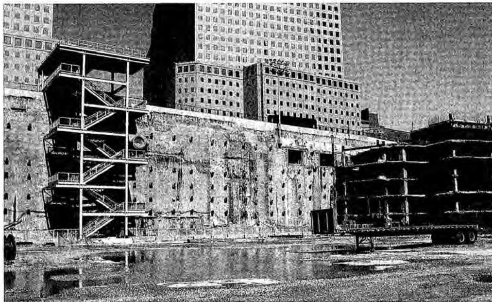
Figure 117. Little to no damage to bathtub, http://911research.wtc7.net/wtc/arch/docs/bathtub_wall1.jpg
