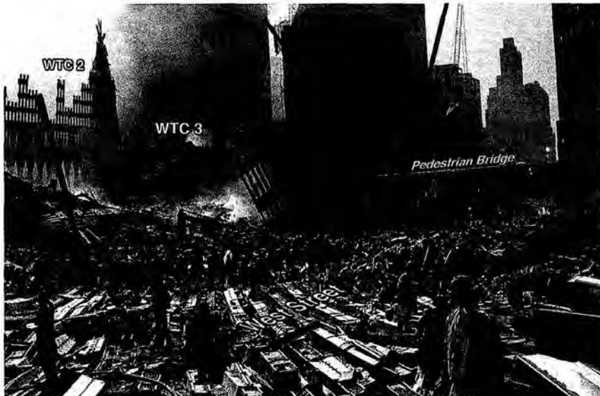
Figure 139. (9/13/01) The West Street laydown of wheatchex.
