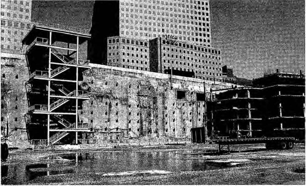
Figure 86. Clearly, the bathtub survived. This is a view from the footprint of WTC1. Notice that the parking structure that was under WTC6 also survived.
