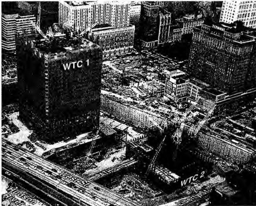
Figure 41. (1970) The below-sea-level bathtub during construction of the WTC.
