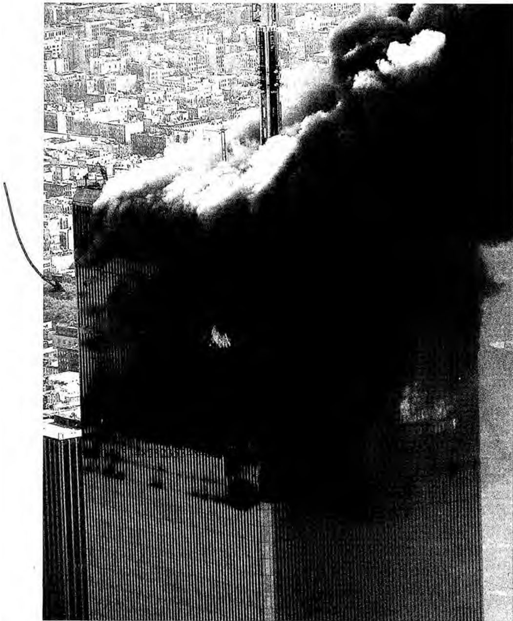
Figure 28. The Western Face of WTC1.
