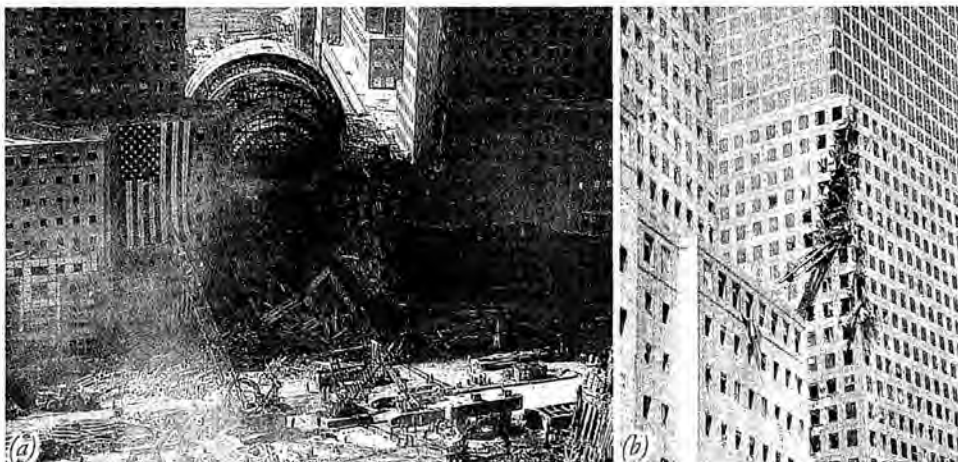
Figure 155. (a) The all-glass Winter Garden had few broken windows, (b) (09/18/01) Damage to WFC3 was no higher than the 18th or 20th floor.
