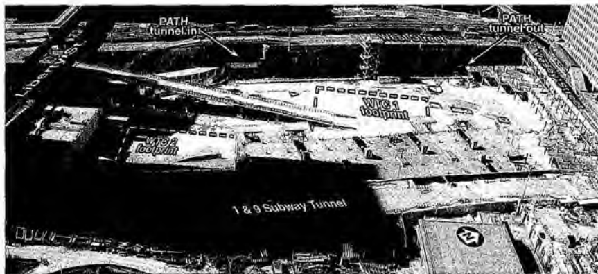
Figure 46. (3/1106) A. composite photo of the bathtub, showing the area below sea level? 1 (combined images) http://i.pbse.com/06/51/57151/1/80214225.ZDLVzNA.IMG_1519.jpg , http://i.pbse.com/06/51/57151/1/80214222.E69PEFED.IMG_1518.jpg .
