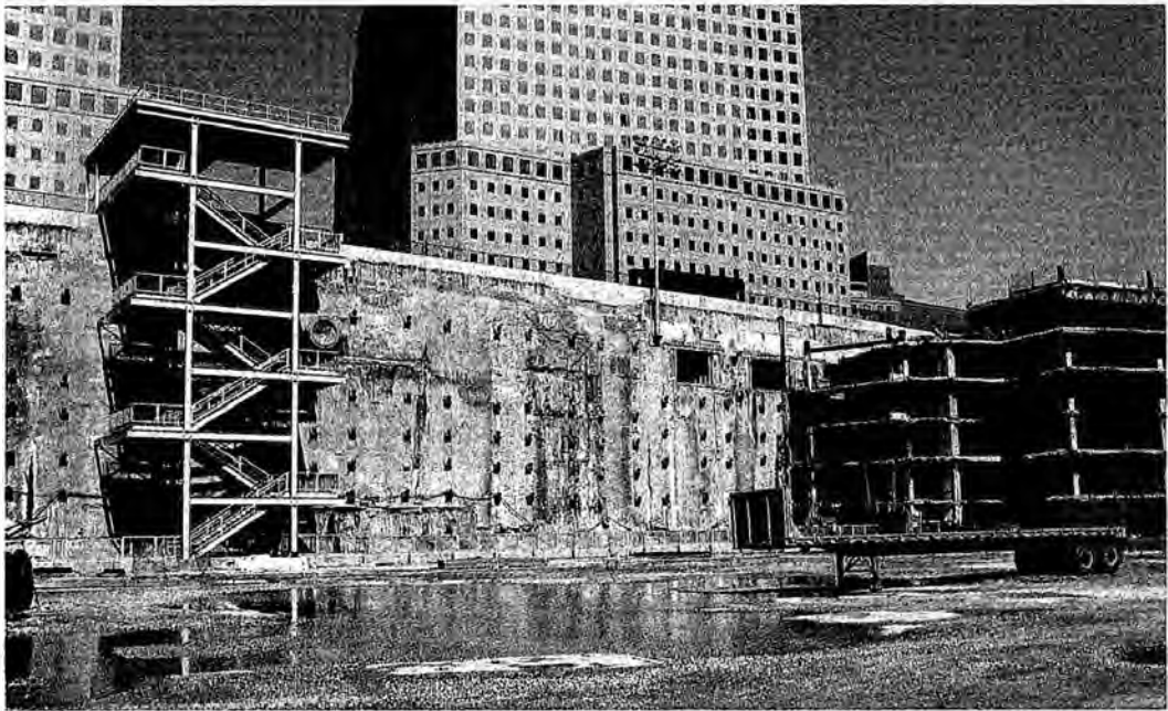
Figure 55. There was no significant damage to the bathtub on 9/11.
