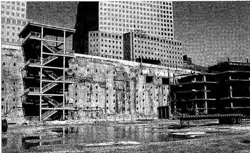
Figure 36. There was no significant damage to the bathtub on 9/11 This picture looks west from the center of the WTC1 footprint,
