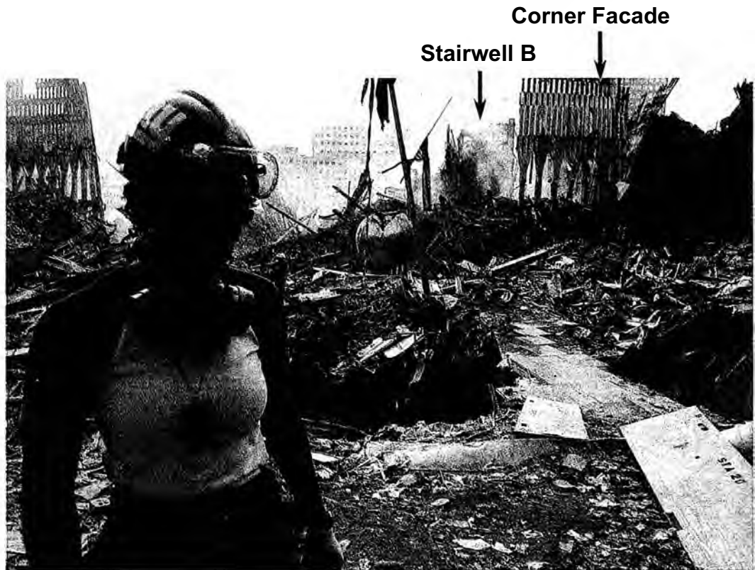
Figure 172. (9/13/01) Looking west through the remains at ground level.
