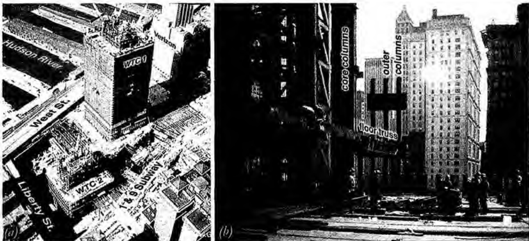
Figure 463. World Trade Center construction with core and structural perimeter of tower.
