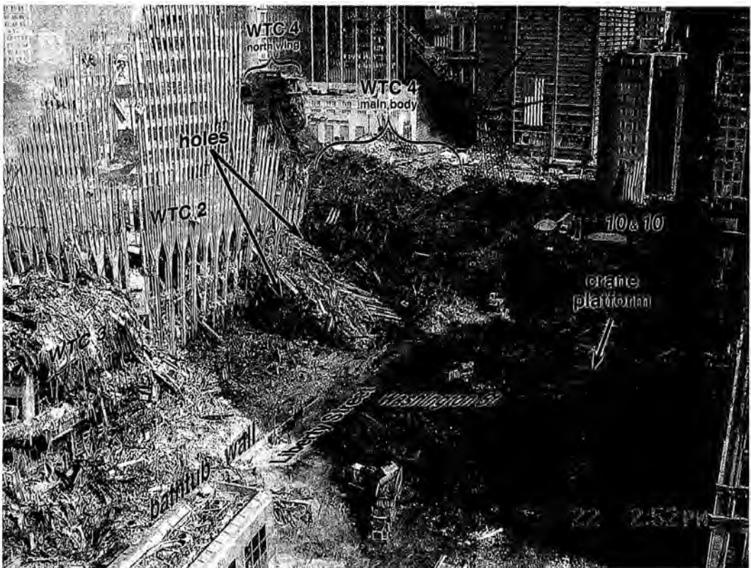
Figure 208. (9/22/01) Holes, missing buildings, and the bathtub wall http://bocadigital.smugmug.com/photos/10698619-D.jpg , http://bocadigital.smugmug.com/
