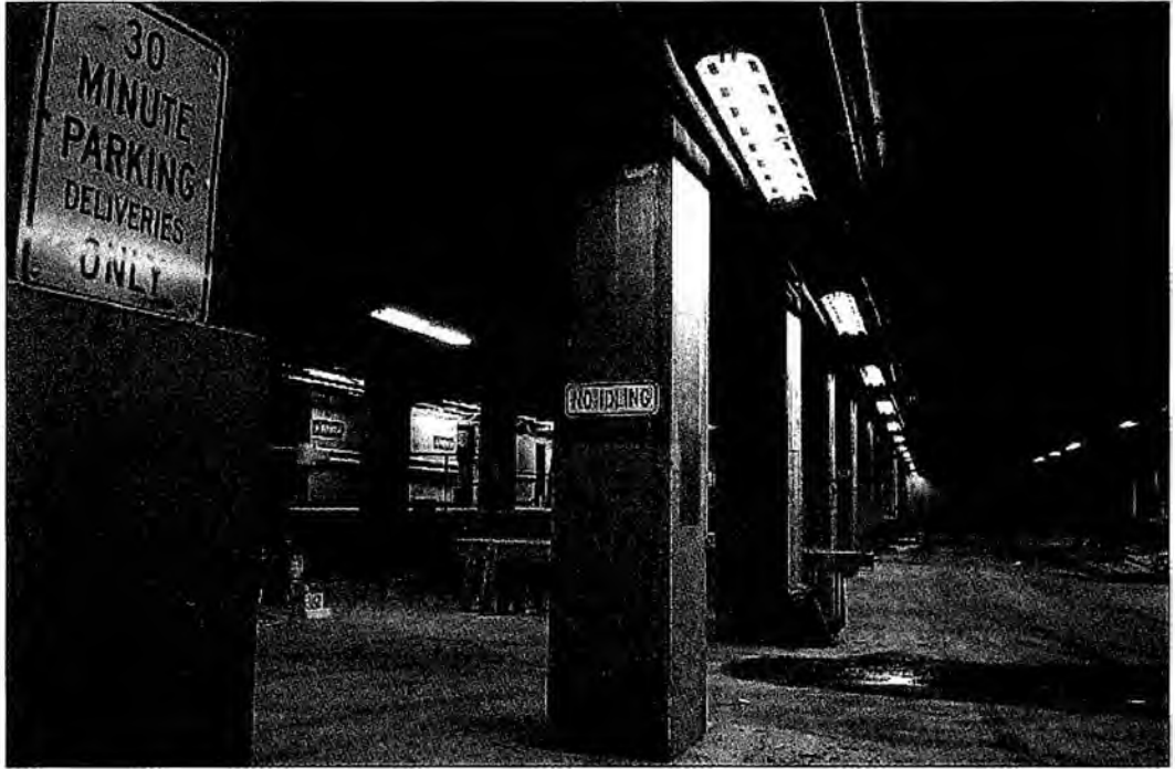
Figure 181. (post 9/11/01) Under WTC4 (green) and WTC5 (purple) from location D, Figure 183. 14 The view is southward, under the WTC mall, where deliveries were made. Figures 54 and 180 are from directly above this green zone near the far end.
