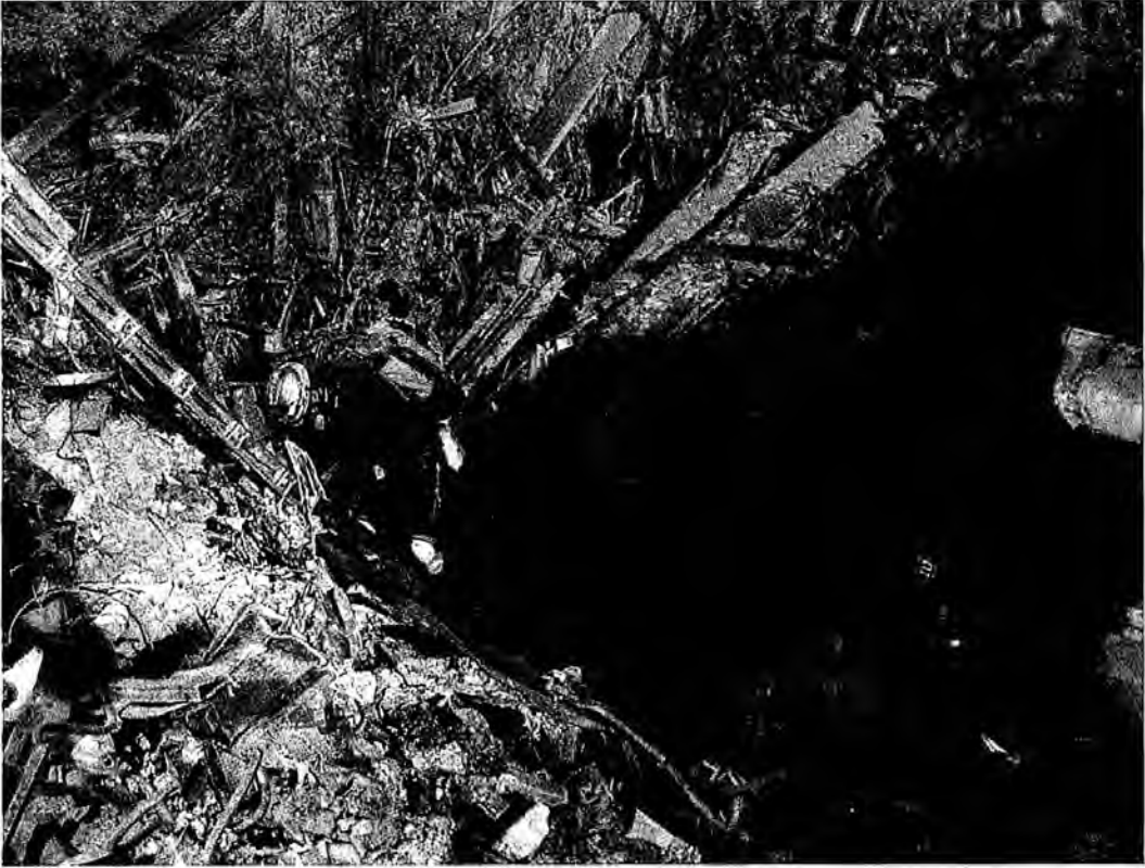
Figure 211. (9118/01) Rescue workers descend into the subbasements below WTC2. (Hole #2) While there is extensive damage, there is little building debris at the bottom of the hole. There is no sign of molten metal. A worker in the distance walks along a massive core column.
