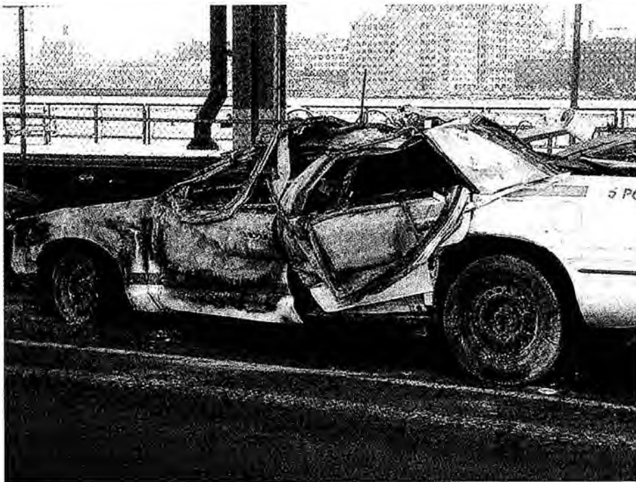
Figure 213. (9/13/01) Peculiar wilting of car doors and deformed window frames of this vehicle found under FDR Drive.
