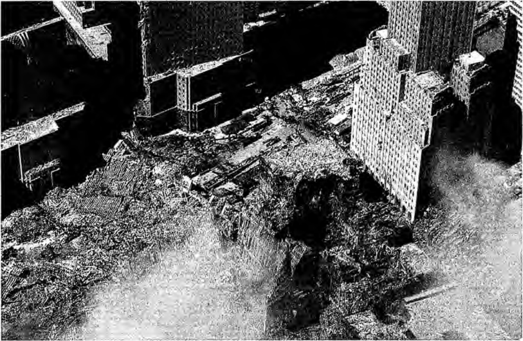
Figure 113. Notice how straight the holes are that cut down through WTC6.
