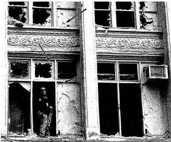
Figure 59. Found holes in windows above the 10 & 10 Firehouse.
