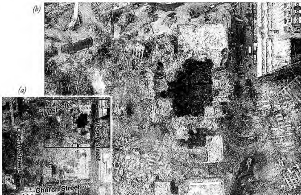
Figure 199. (9/23/01) This shows the vertical cutouts in the center of WTC6. To the left of WTC6 are the remains of WTC1. Note the fairly consistent diameter of the holes. The holes are essentially empty: little debris visible inside the holes. (NOAA) 1
