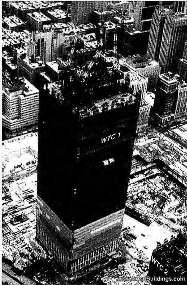
Figure 492. World Trade Center construction of core and structural perimeter, http://data.GreatBuildings.com/gbc/images/cid_wtc_myw_WTC_const.3.pg 15
