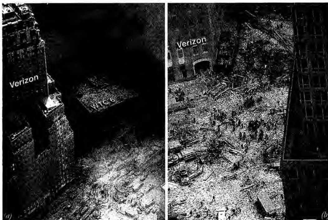
Figure 128. Photos taken in the afternoon of 9/11/01 before WTC7 was destroyed, (a) Looking southeast toward WTC6, across the West Street and Vesey Street intersection, (b) closer, (view A, Figure 127) (a) http://11wtc.freehostia.com/gallery/originalimages/GJS-WTC131.jpg , (b) http://911wtc.freehostia.com/gallery/originalimages/GJS-WTC132.jpg .
