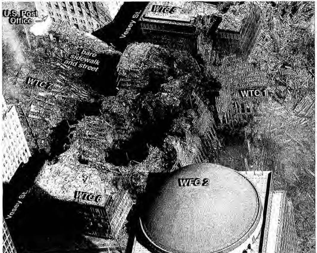
Figure 19. A view over the dome of WFC2 shows the damage to WTC6 in the center of the photo. To the left is the collapsed WTC7. Its debris stack is about five stories high. To the right of WTC6 is the remaining north wall of WTC1, which leans toward WTC6, an eight-story building. Where did the wall go? Where did the top 102 floors of the north wall go? They did not fall on WTC6 or WTC7 because there are no steel "wheatchex" outer cladding there. Some of the core of WTC1 remains, but where is the rest of the core? The amount of steel on the ground barely covers the ground. If there is no wheatchex debris from WTC1 piled on top of WTC6, how did WTC6 get cored out from the top down?!
