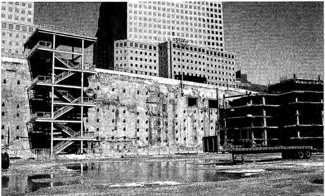
Figure 194. The western bathtub wall above continued to hold back the Hudson River after 9/11 with no significant damage. This is a view from within the WTC1 footprint.
