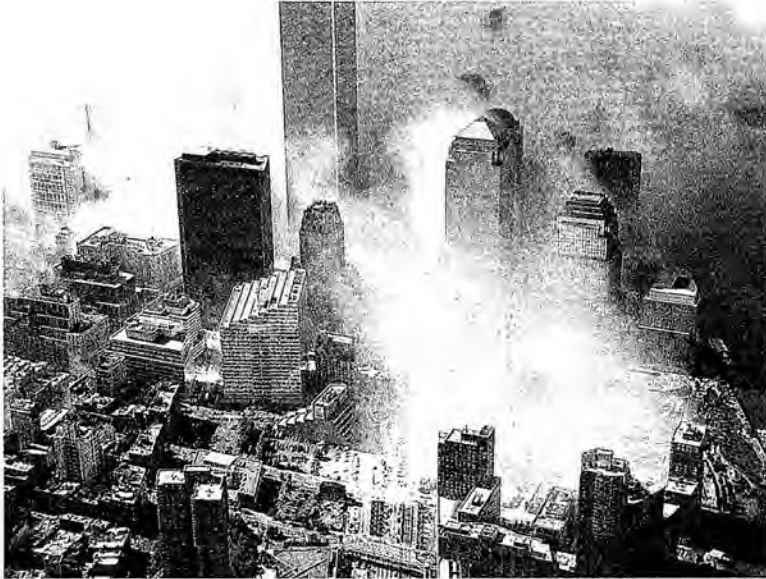
Figure 322. After the dust rollout of WTC2.
